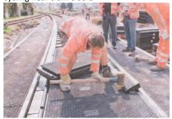
pros and cons of 'VeloSTRAIL track filler devices at pinch points, as used in Germany
